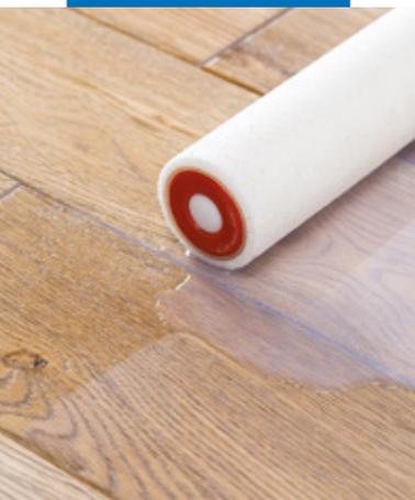
After sanding application of Ultracoat two-component, water-based varnish
