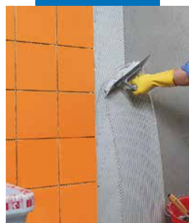
Bonding of ceramic covering over MapeWall Render & Strengthen
