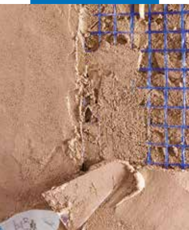
Application of the second layer of MapeWall Render & Strengthen
