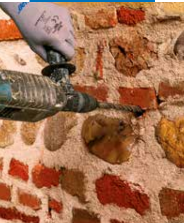
Preparing the holes for Mapenet EM Connector
