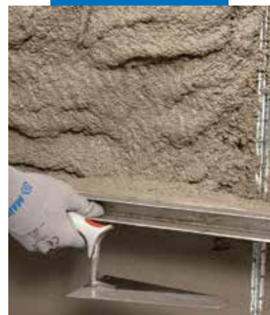
Levelling MapeWall Render & Strengthen with a straight-edge
