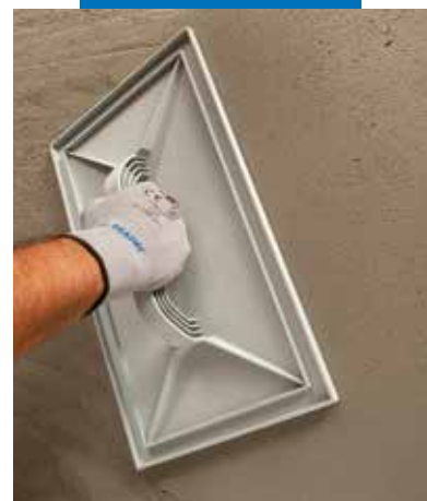
Levelling the substrate
